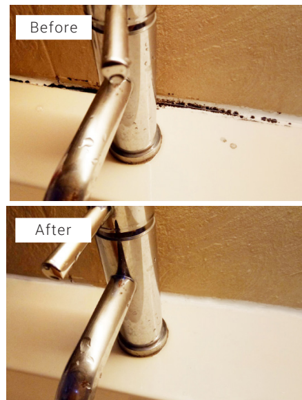
MOULD ON KITCHEN SINK
