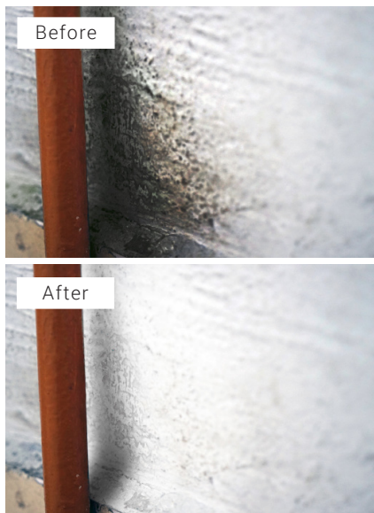
MILDEW ON WALL
