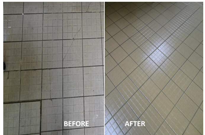
Diamond Restoration on Ceramic Floor
